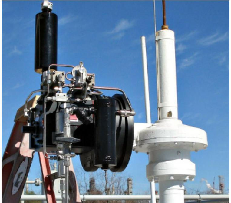
ATI gas motor actuators utilize unregulated pipeline gas to provide a simple, reliable and economical means of automating valves without gear boxes. Using pipeline gas up to 1500 psi to drive a gas motor coupled to a gear train, these actuators motorize the input shaft of the valve gear box. Instead of spending 30-45 minutes operating a gear box hand wheel, the gas motor actuator can open or close a 36-inch valve in less than two minutes.
