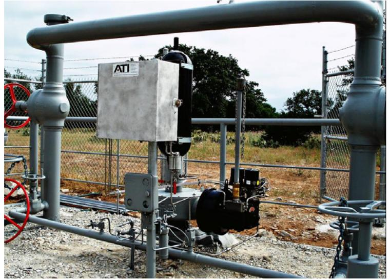
The Gevalco Automatic Line Break Control module from ATI is designed to automatically close main pipeline valves in the case of a major leak or break. By quickly and reliably closing the main pipeline block valves, gas loss can be minimized to prevent fires and other catastrophic disasters.
